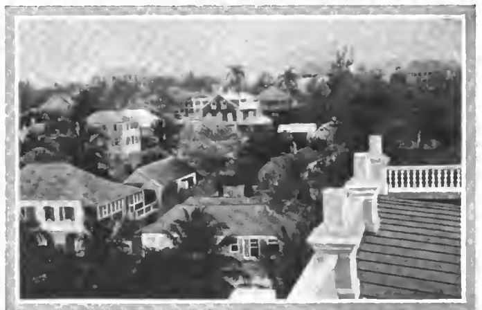
GENERAL VIEW OF TOWN SHOWING GOVERNOR'S PALACE
